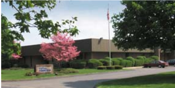
Total Communications' Main Office in East Hartford, CT
